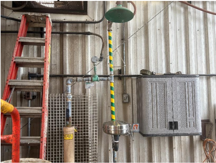
Figure 21: New Eyewash Station in Lime House No. 3
