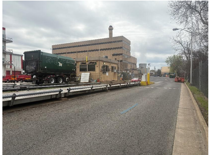
Figure 8: Scale House in Operation
