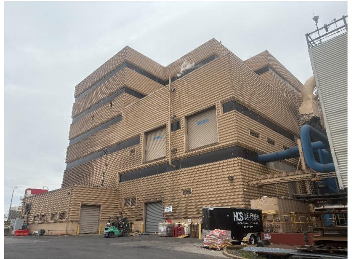
Figure 2: North Side of Facility - Siding Half Pressure - Washed
