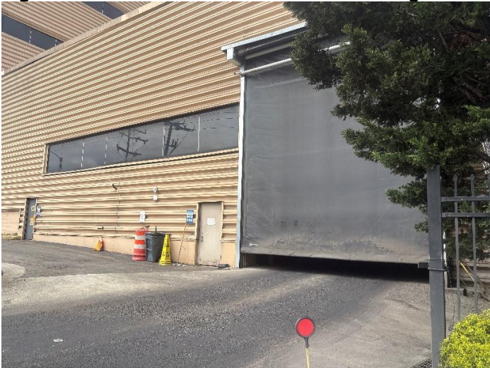
Figure 9: Tipping Floor Door in Operation
