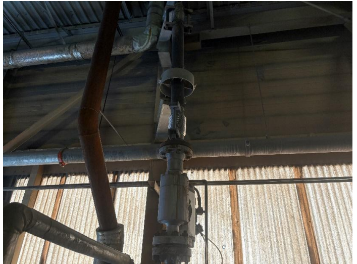
Figure 20: New Expansion Joint on North side of Boiler No. 1
