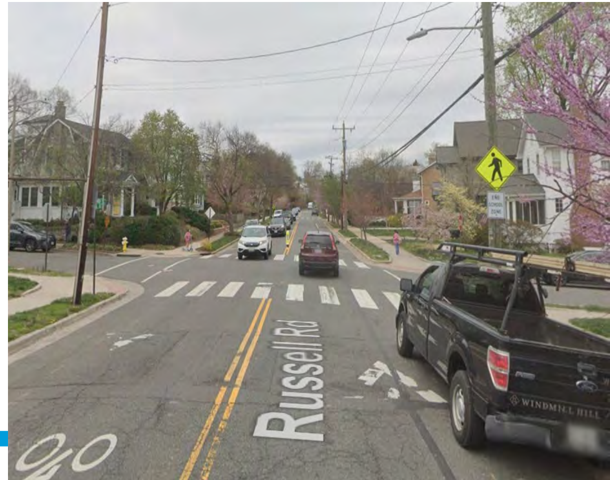
Parked vehicle blocks sight of curb ramp
