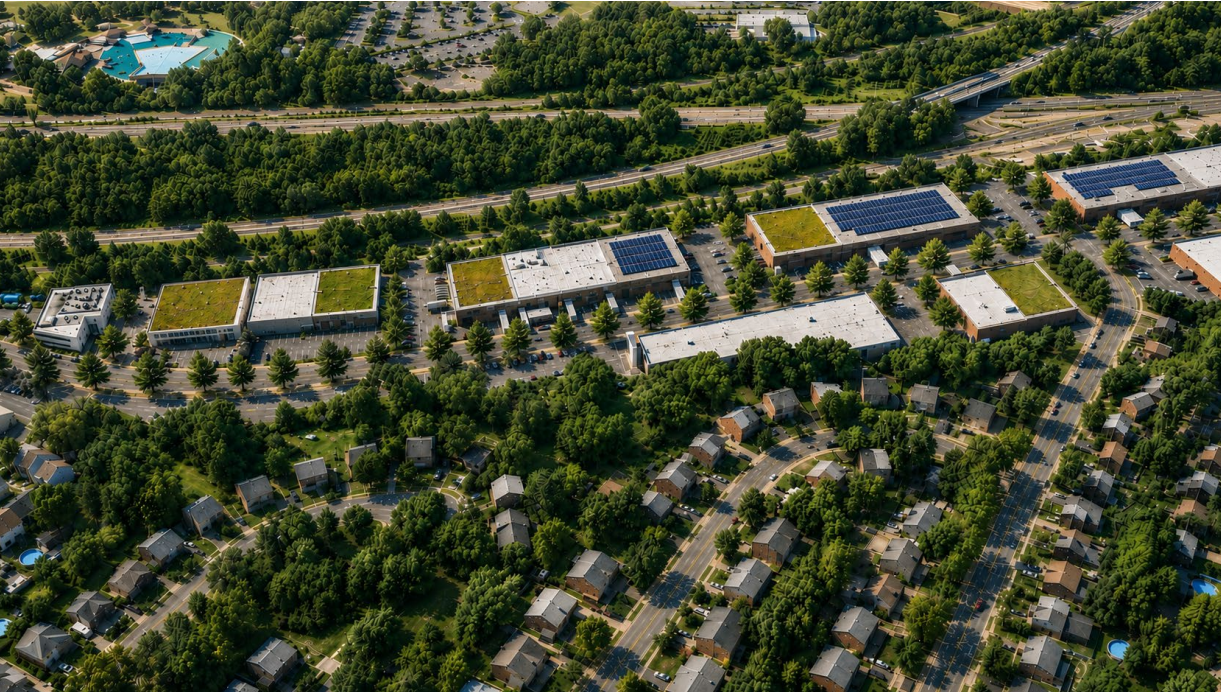
Depicted (Left): Large-scale solar panels on existing Wheeler Avenue warehouse roofs – opportunities to make existing buildings more energy efficient.
