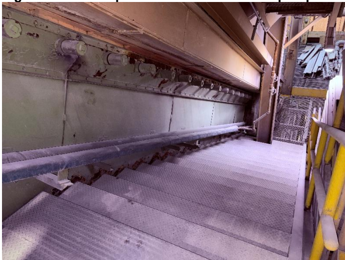
Figure 9: Stairwells between boilers – no issues observed
