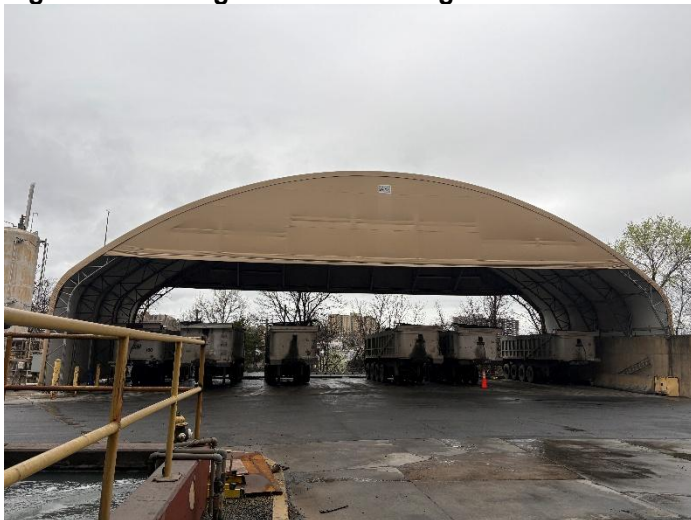
Figure 3: Ash trailer canopy in good condition
