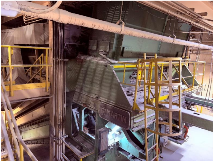
Figure 13: Boiler No. 3 transition chute holes repaired
