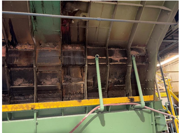
Figure 14: Plate repairs made to Boiler No. 1 feedchute - painting should be completed
