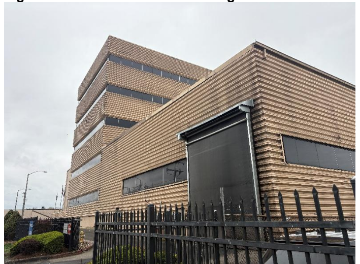
Figure 6: Tipping Hall exit door in good condition
