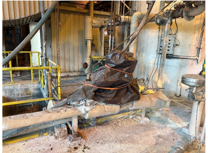
Figure 2: Tarp wrapped around settling basin pump
