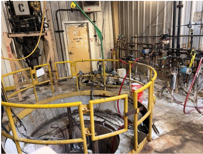
Figure 21: Unit 3 SDA Penthouse general condition – no issues observed
