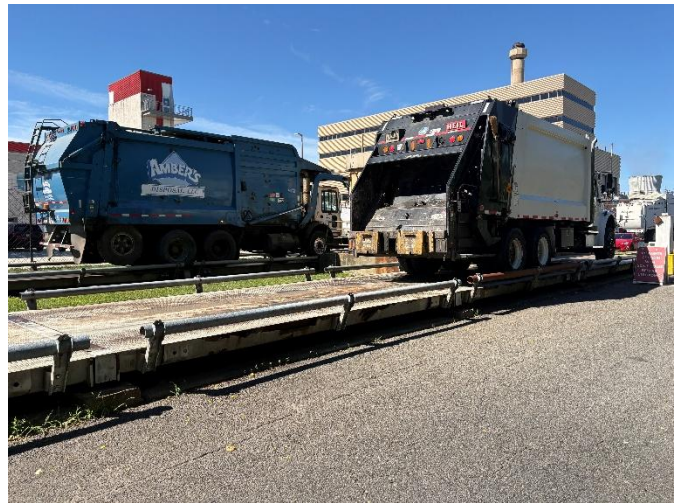
Figure 2: Deficiency Item 0326-02: Side bar of truck scale repaired
