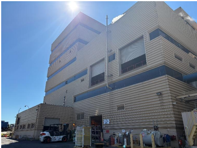
Figure 1: North side of facility clear of debris and no siding discoloration
