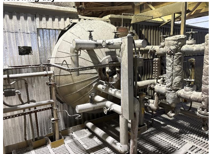
Figure 12: Deficiency Item 0221-1: New lagging around Boiler No. 3 steam drum
