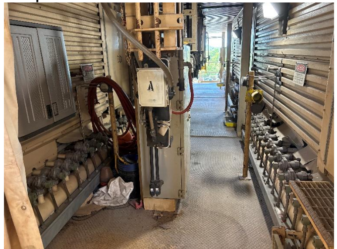
Figure 16: General housekeeping of Unit 2 baghouse area
