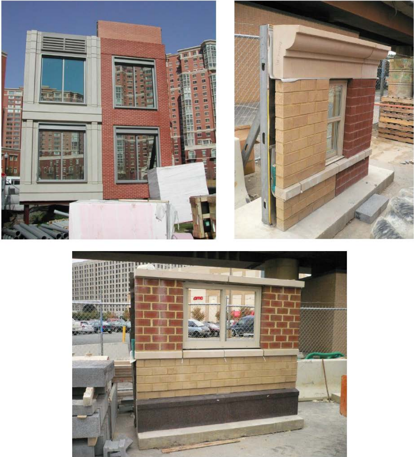
ATTACHMENT 2: EXAMPLES OF CONSTRUCTED MOCK-UP PANELS
