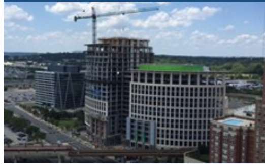
2401 Eisenhower ave worksite
