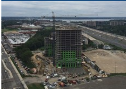
750 Port street worksite
