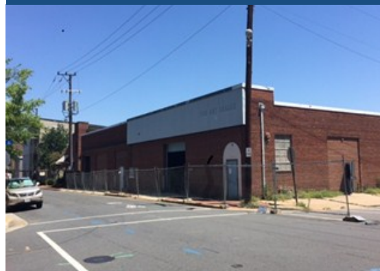
220 S. Union Street worksite
