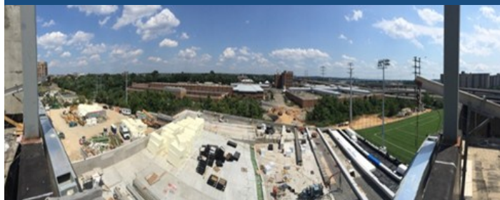
1820 Limerick street worksite
