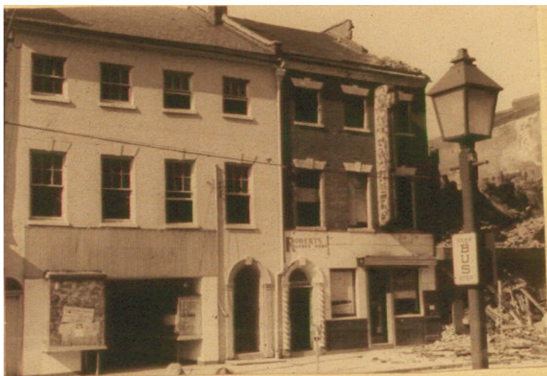
Fig. 4: Adam Lynn's house on the left, before demolition, 518-522 King St. (ALEXANDRIA ARCHAEOLOGY COLLECTION).
