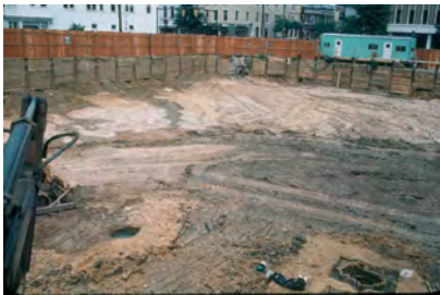
Fig. 1: The construction site, 1977 (ALEXANDRIA ARCHAEOLOGY COLLECTION)
