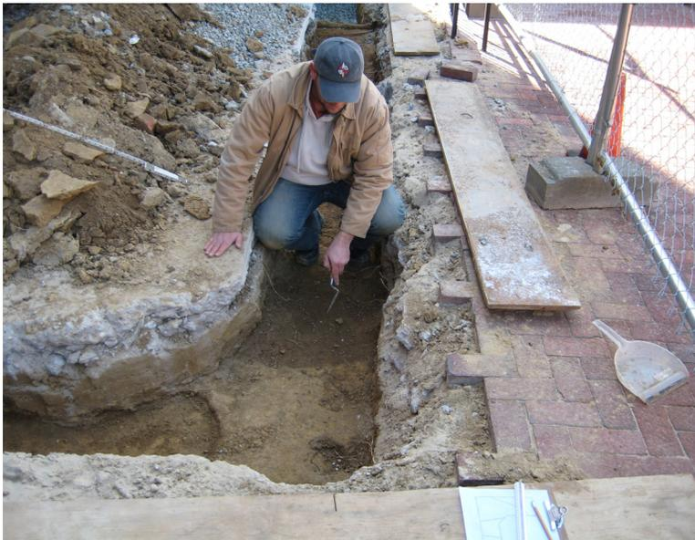
In order to avoid disturbing these probable graves, excavation of the foundation trench was halted at that depth. The trench was then filled in with gravel and reinforced concrete, so it will serve as the foundation of the ramp. The Parish Hall will become more accessible to the whole church community, and the historic graves have been preserved intact.
