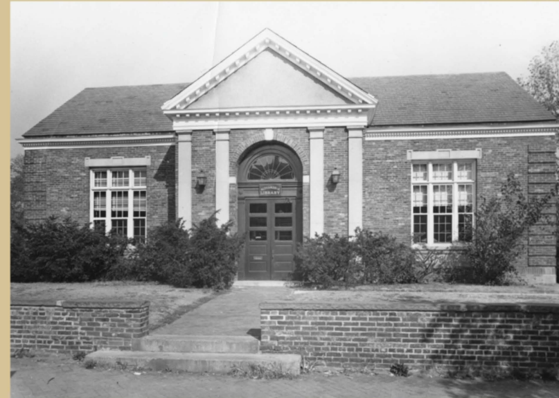
Picture of the new Barrett Library taken in the late 1930s. The building has been expanded over the years.
