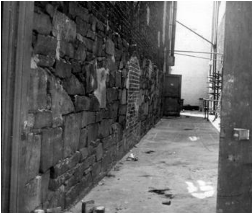
203 South Strand, wall before renovation Credit: Alexandria Library - Local History/Special collections
