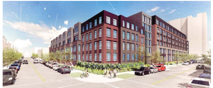
View at the corner of Pendleton Street & N. Royal Street
