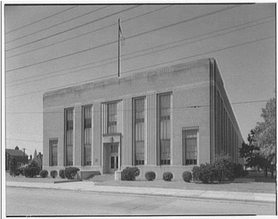
Figure 10: "Chesapeake and Potomac Telephone Company. C&P building at 1306 Mt. Vernon Ave., Alexandria, Va." Theodor Horydczak, photographer. September 1947. Courtesy of the Library of Congress Prints and Photographs Division Washington, D.C. Accessed 5 May 2014 at http://www.loc.gov/pictures/item/thc1995005729/PP/
