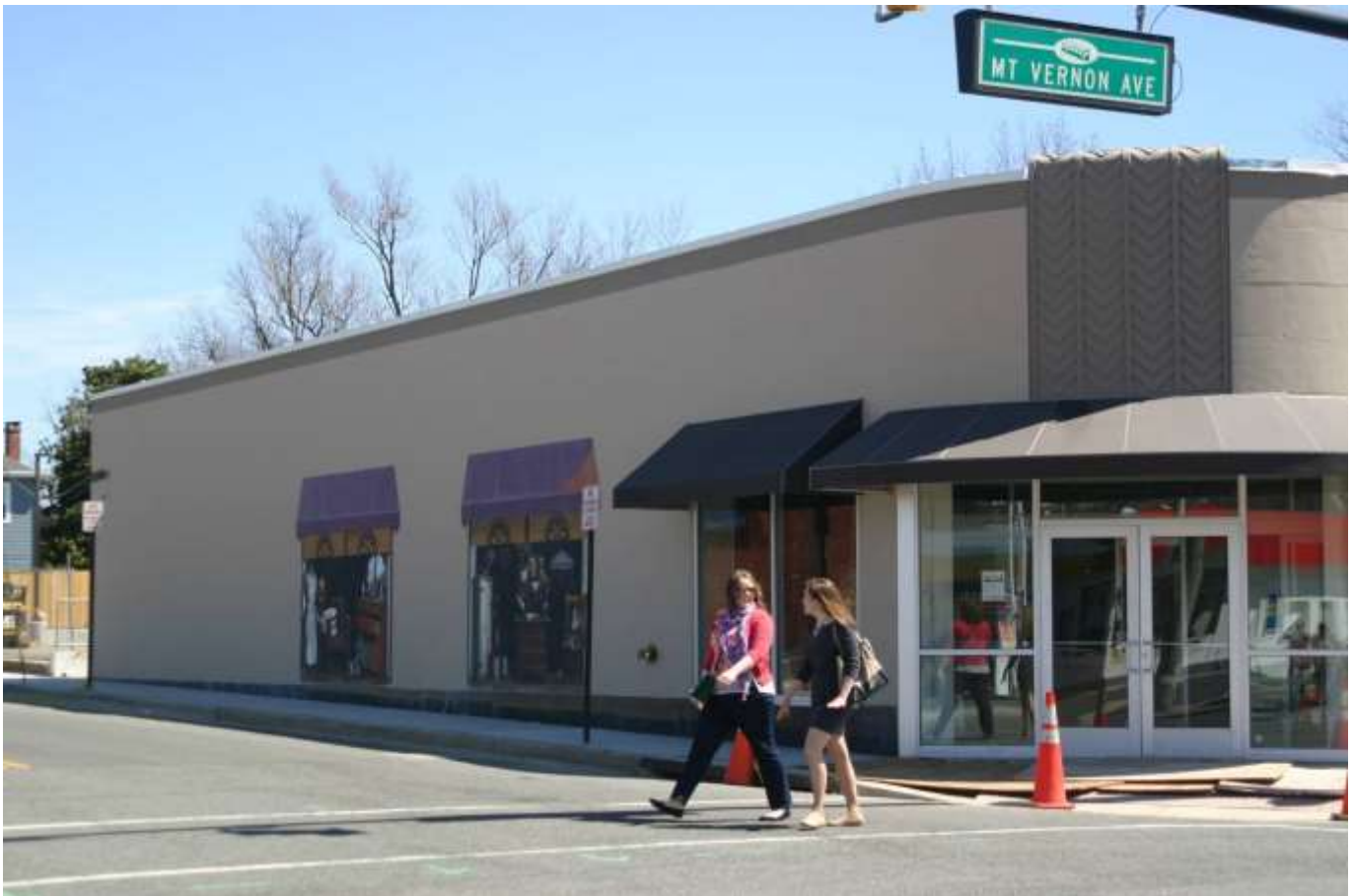
4. 1509-1517 Mt. Vernon Avenue. North elevation, oblique angle, facing 131° SE. Photograph by Gwen White, 4/6/14. 12/22/2015
