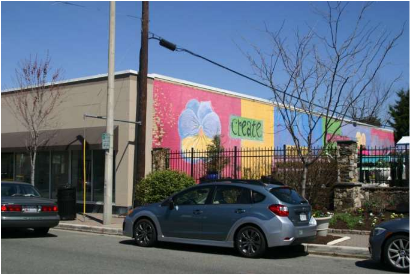
5. 1509-1517 Mt. Vernon Avenue. South elevation, oblique angle, facing 40^{\circ} NE. Photograph by Gwen White, 4/6/14.
