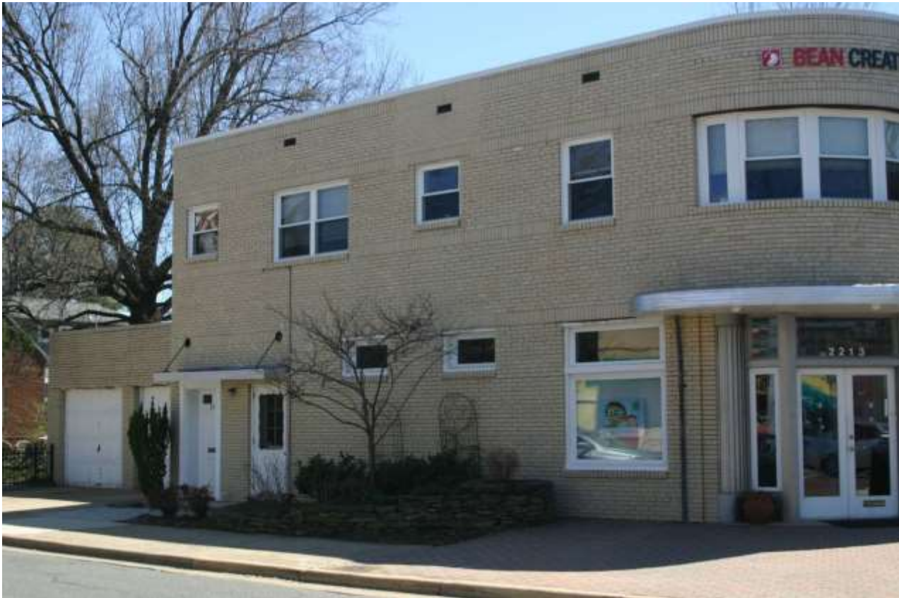
3. 2213 Mt. Vernon Avenue. North elevation, oblique angle, facing SE. Photograph by Gwen White, 4/6/14.
