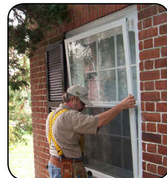
Installation of an exterior storm window.
