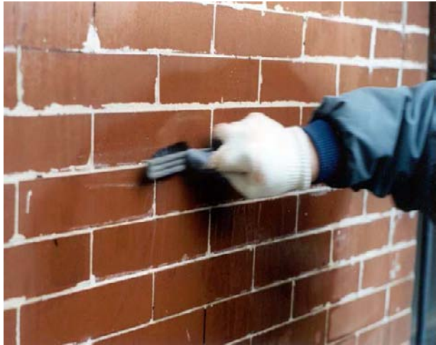
Fig 4. Scrub away the stains and mortar residue using a brush with nylon or natural bristles.
