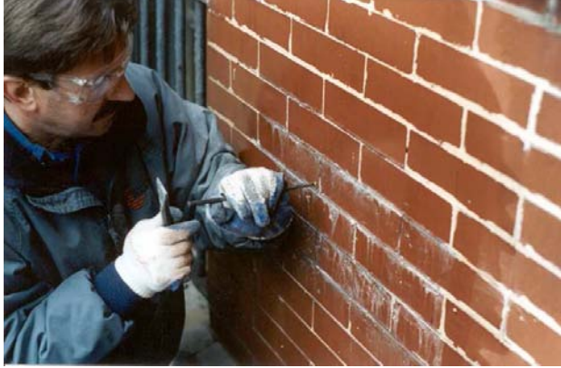
Fig 9. After the center of the mortar joint has been cut, use hand tools to carefully remove mortar from the sides of the brick.
