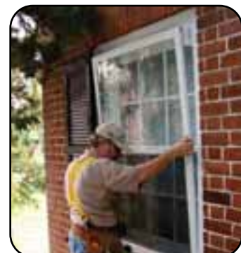
Installation of an exterior storm window.
