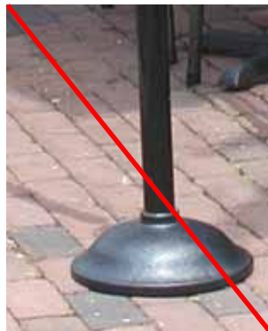
FIGURE 5 Domed stanchion bases are not permitted
