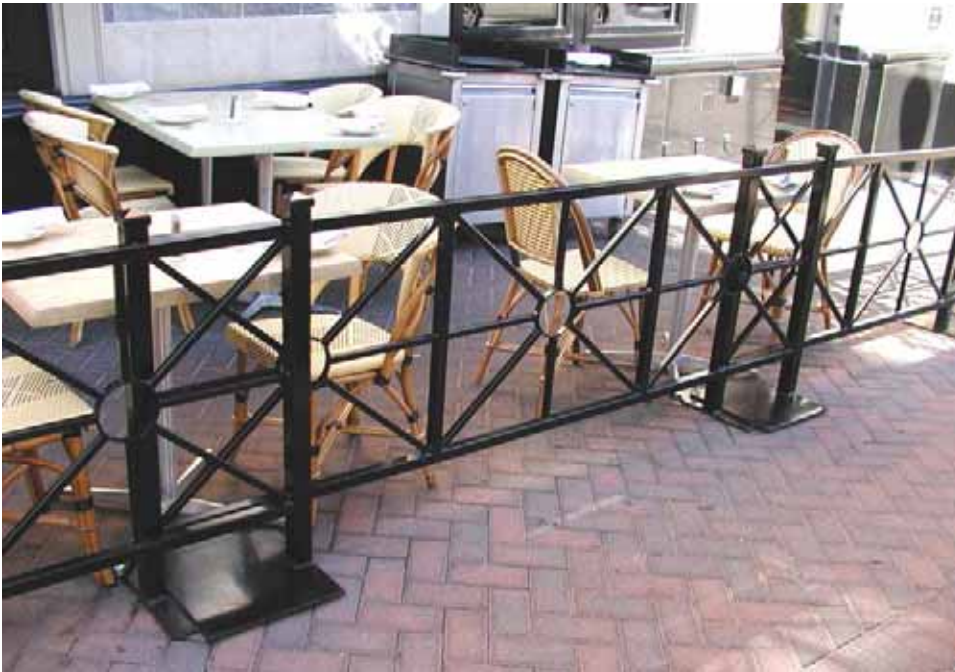
FIGURE 6 Acceptable sectional fencing design: freestanding
