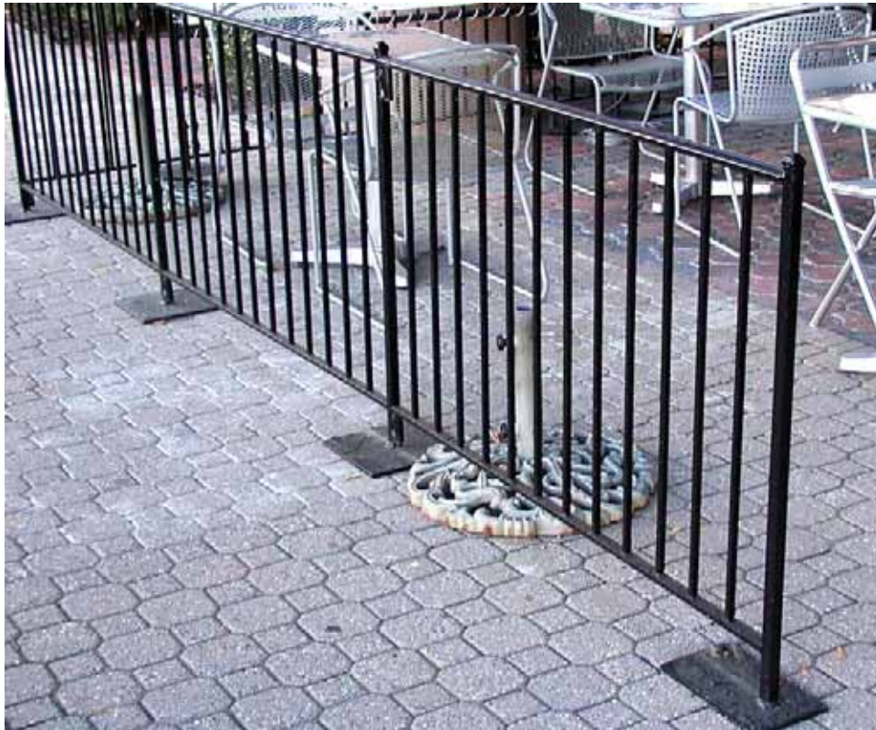
FIGURE 2 Acceptable sectional fencing design
