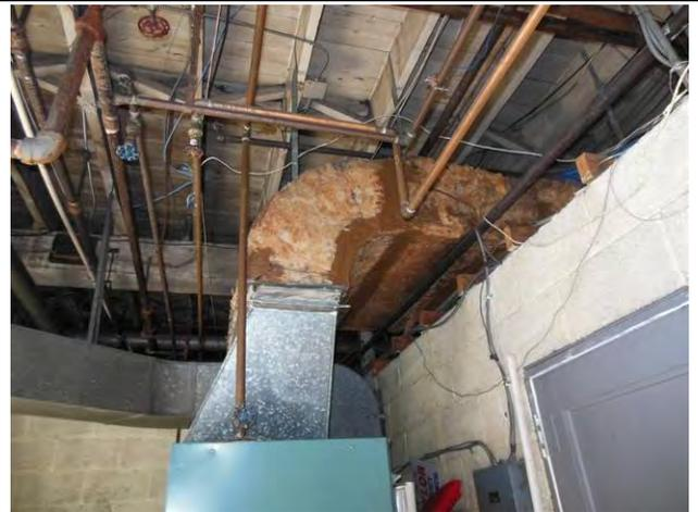
4. View of the brown duct mastic and white vibration cloth, Samples 4-9.
