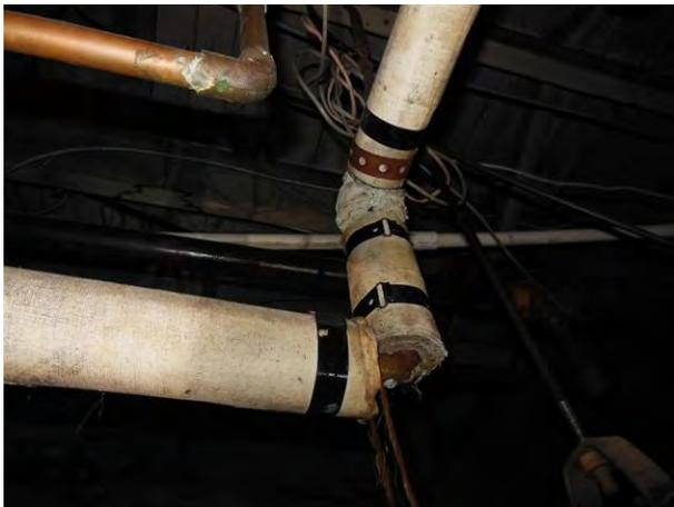
5. View of pipe insulation and hard elbow insulation, Samples 10-15.
