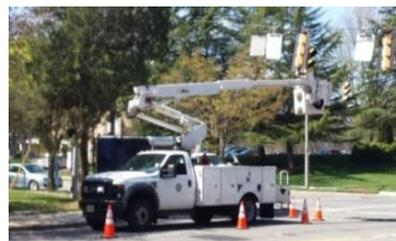
**Traffic Lights LED Replacement Program** – The City replaced all 2500 incandescent traffic lights with energy efficient LED lights. This reduces energy consumption by 650,000 kWh and \$70,000 in electricity costs annually. As a pilot project using a US Department of Energy grant, City also installed 34 **LED street lights** in partnership with Dominion Virginia Power. Currently, new developments in the City are required to install LED street lights.
