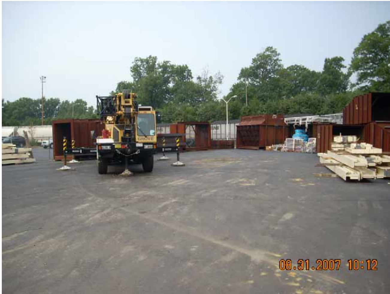
Equipment staged in northwest parking lot.
