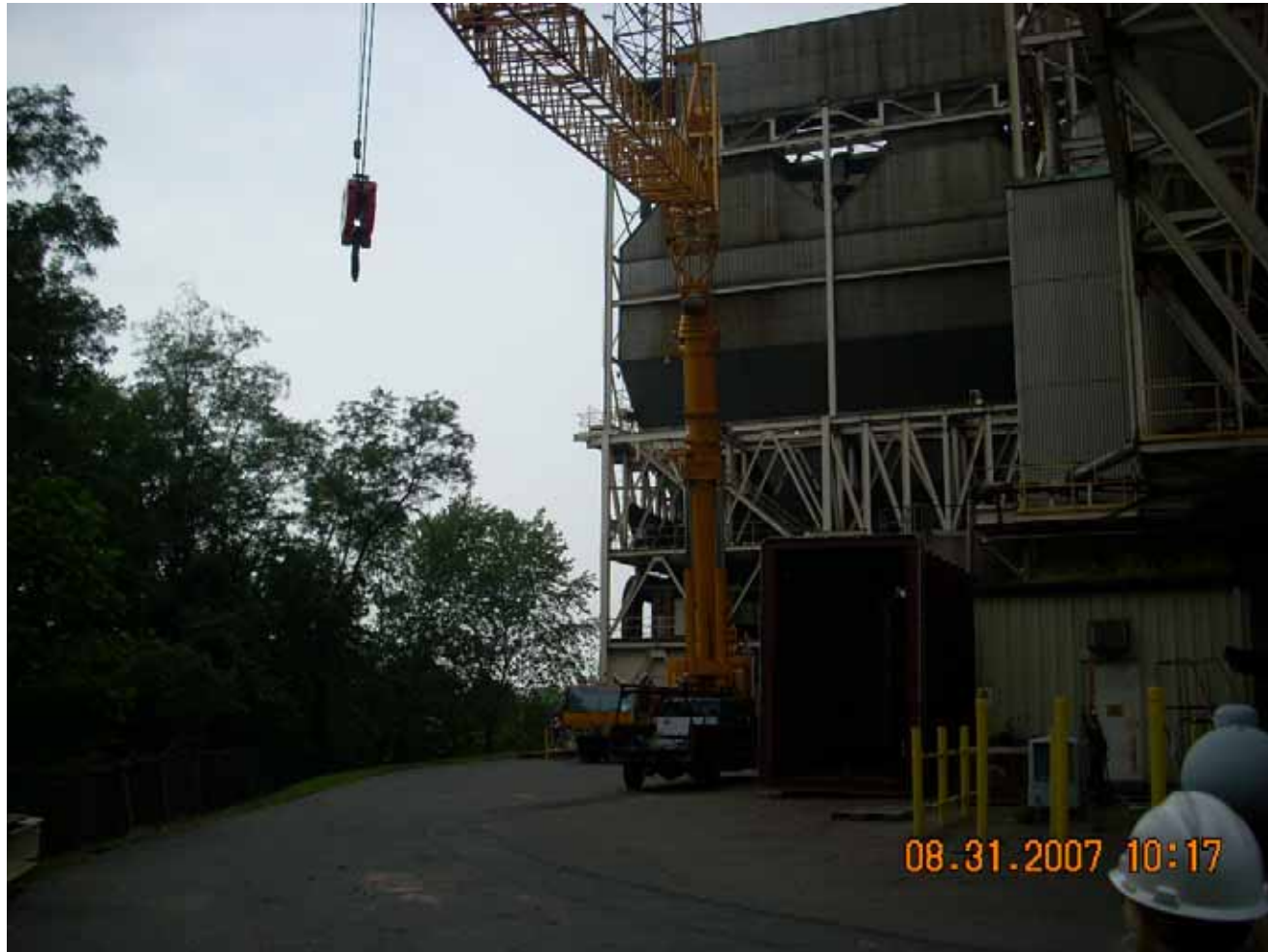
Large crane (not in use at the time of the site visit) staged on the northeast side of the plant.
