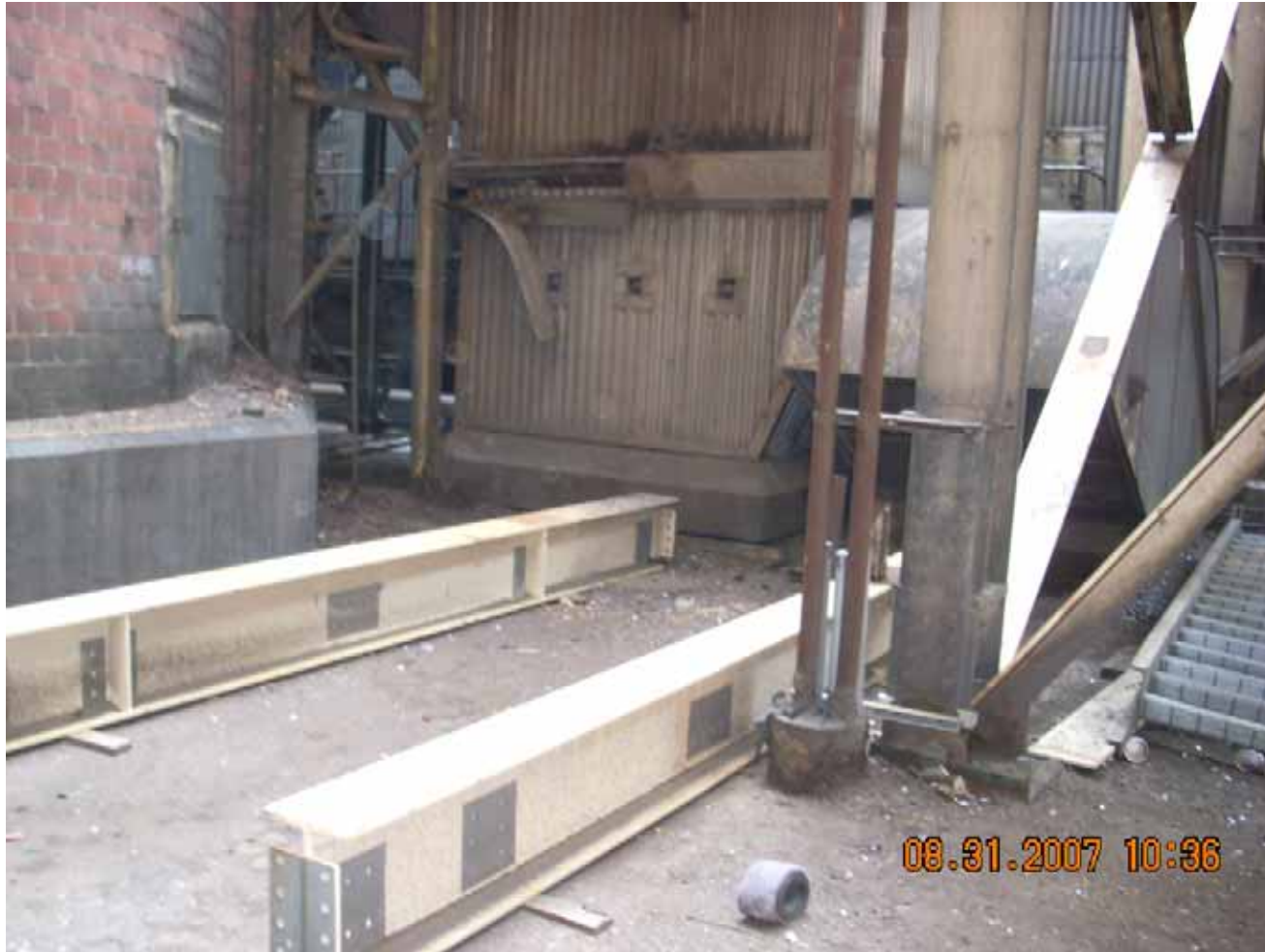
Structural beams and stairways removed near base of Stack #2.
