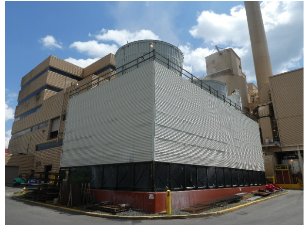
Photo: Cooling Towers
