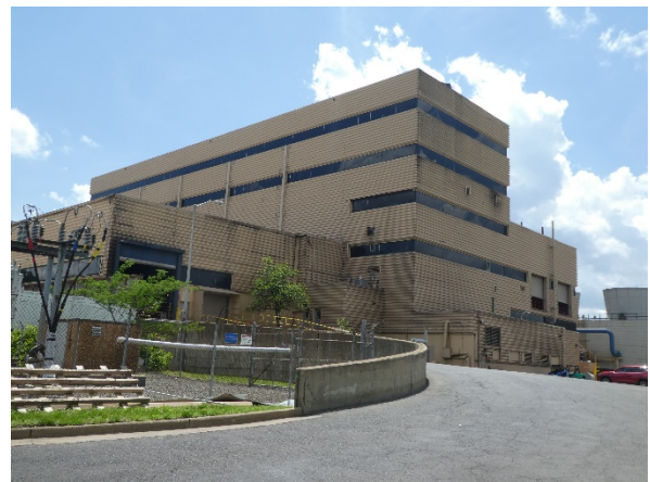
Photo: North Side of Facility and Tipping Floor Entrance
