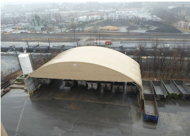
Photo: Ash Trailers and Canopy
