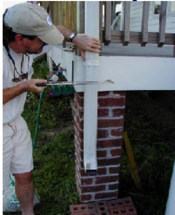
**Step 5.** Put the barrel in place, with the top ring and mosquito screening on top. Re-attach the curved downspout end-piece to the downspout.
