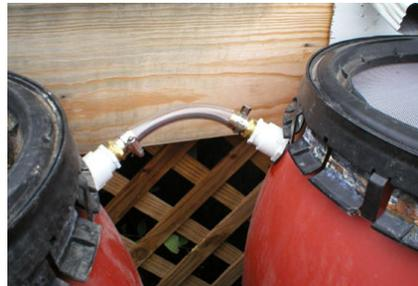
There are many ways to connect one barrel to another. Here, we used some plastic tubing and hose clamps.
