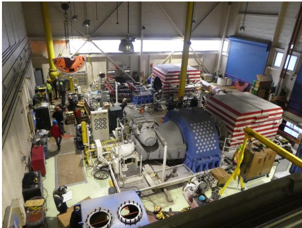
Photo: Turbine Generator No. 1 Major Overhaul in Progress – November 2019
