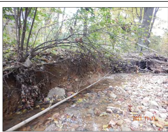
Figure 22. Stream Reach #2 – Looking Downstream (Station 2+20)
