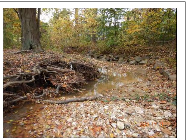
Figure 4. J-Hook Vane #1 – Looking Downstream (Station 2+20)
