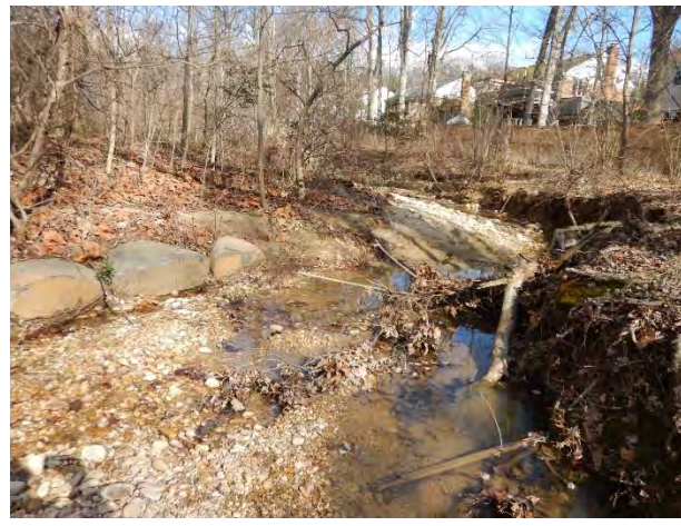
Figure 32. J-Hook Vane #1 Looking Upstream (Station 1+90, January 2021)
