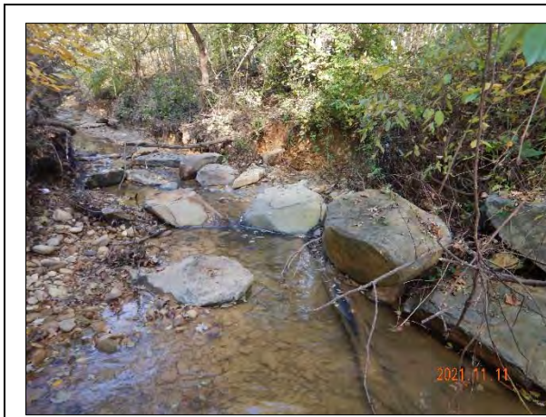
Figure 11. J-Hook Vane #3 – Looking Upstream (Station 4+20)
