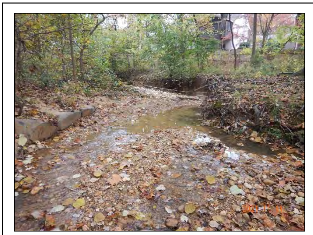
Figure 3. J-Hook Vane #1 – Looking Upstream (Station 1+70)
