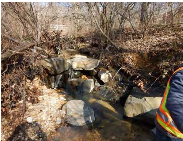
Figure 35. J-Hook Vane #3 (January 2021); Duplicate Image for Reference
