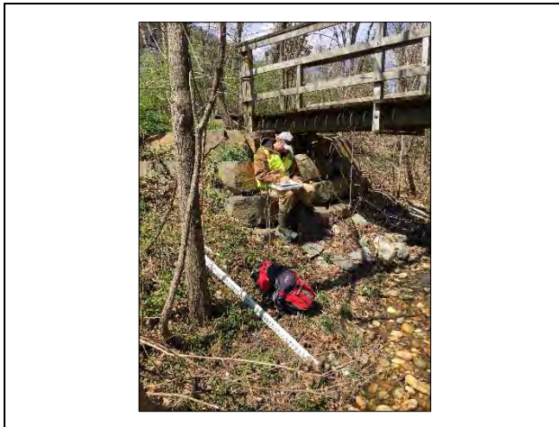
Figure 13. Right Bridge Abutment – Looking Upstream (April 2018, Station 5+00)
