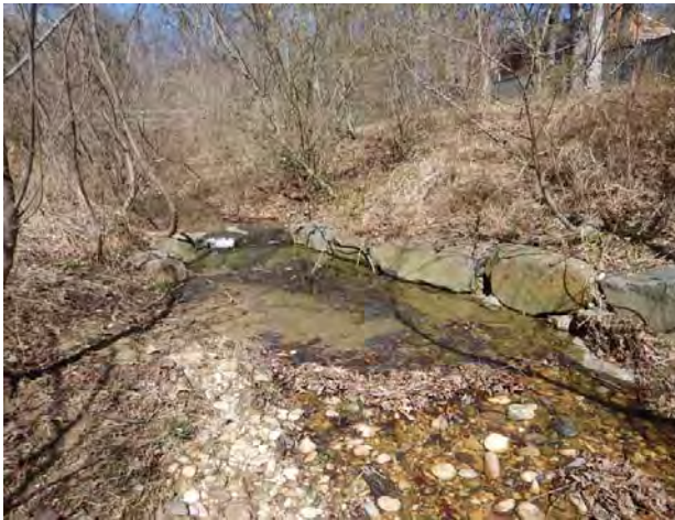
Figure 33. J-Hook Vane #3 (Station 4+20, March 2018)
