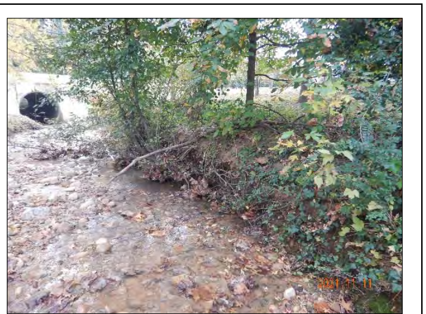
Figure 20. Stream Reach #1 – Looking Downstream (Station 0+50)
