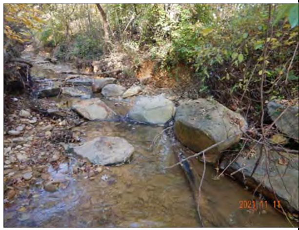
Figure 36. J-Hook Vane #3 (November 2021)
