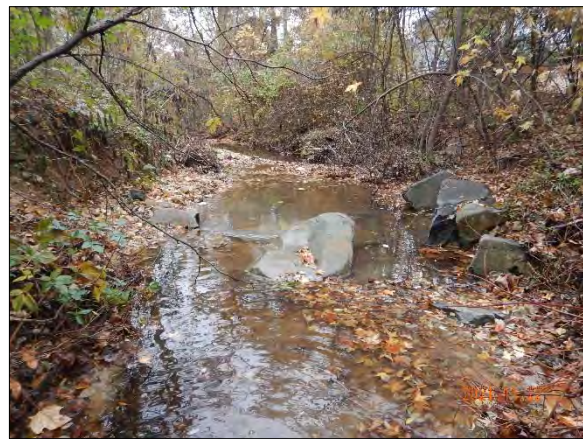
Figure 10. J-Hook Vane #2 – Looking Downstream (Station 3+80)
