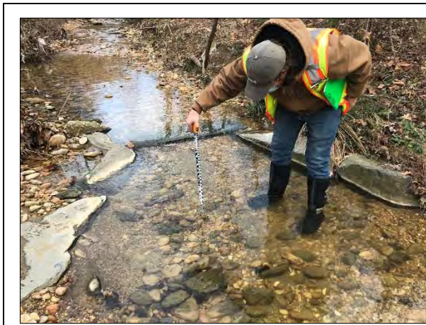
Figure 7. Cross-Vane #1 – Looking Upstream (January 2021, Station 2+40)
