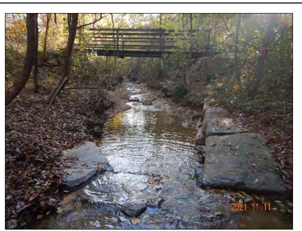
Figure 16. Cross-Vane #2 – Looking Downstream Towards Bridge (Station 5+50)
