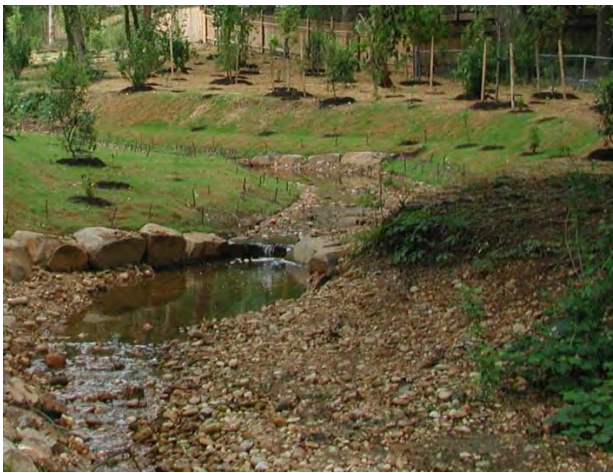
Figure 31. J-Hook Vane #1 As-Built Looking Upstream (Station 1+90, 2010)
