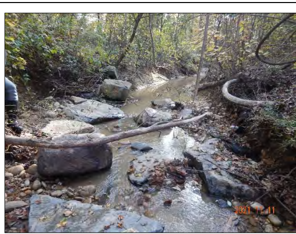
Figure 12. J-Hook Vane #3 – Looking Downstream (Station 4+30)
