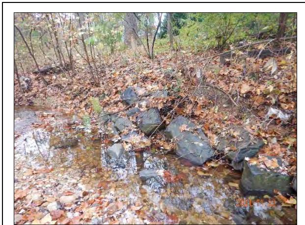
Figure 5. Rock Toe Looking Downstream (Station 1+60)
