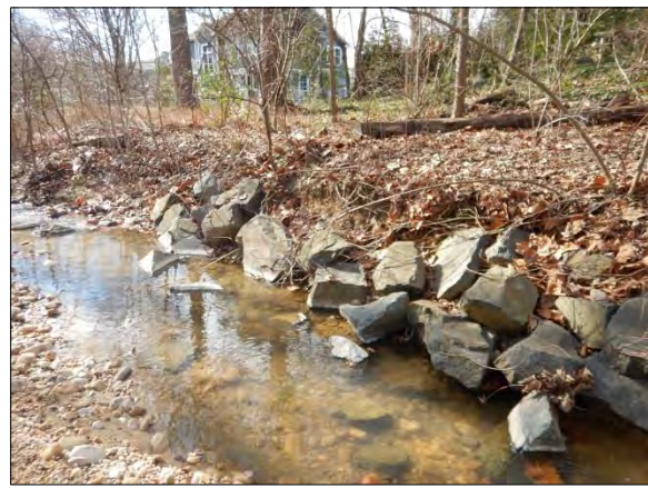
Figure 75. Rock Toe (Station 1+60)
