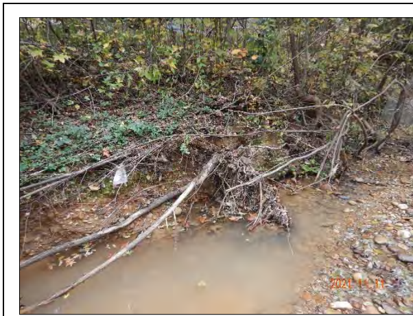
Figure 23. Stream Reach #3 – Looking Upstream Right Streambank (Station 3+30)
