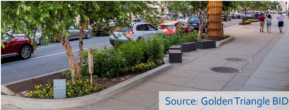
Rain gardens/stormwater features
