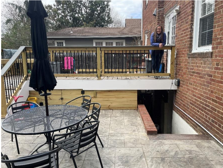
Kelsey Davis, Alexandria resident, shows City staff the flood mitigation improvements done to her house. (City of Alexandria)
