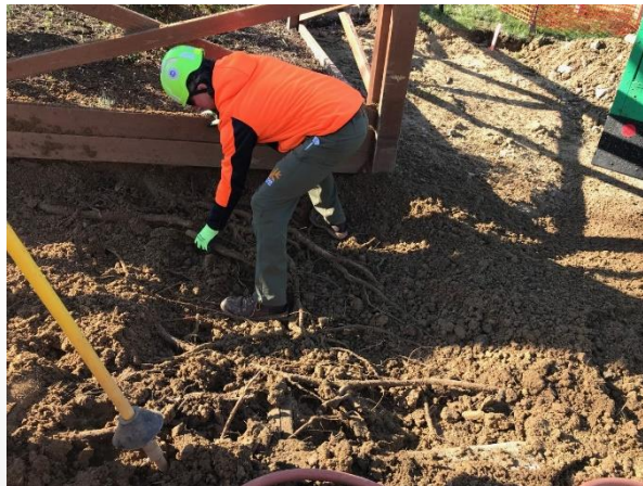
Air spading may be used to loosen compacted soil, to expose tree roots, and to keep critical root systems intact. This application was used for construction of a sidewalk at Ewald Park.
