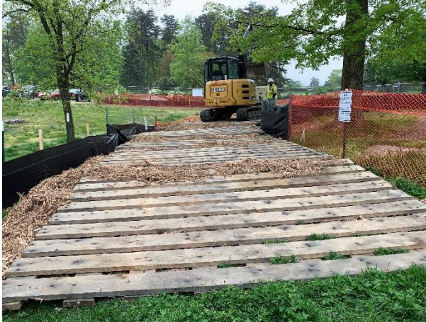
Tree mats were used for equipment access during construction of the Fort Ward picnic shelter pathway
