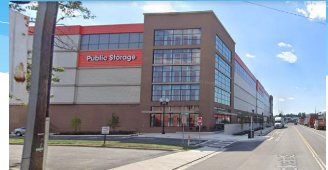
Recent industrial building constructed on Pickett Street
